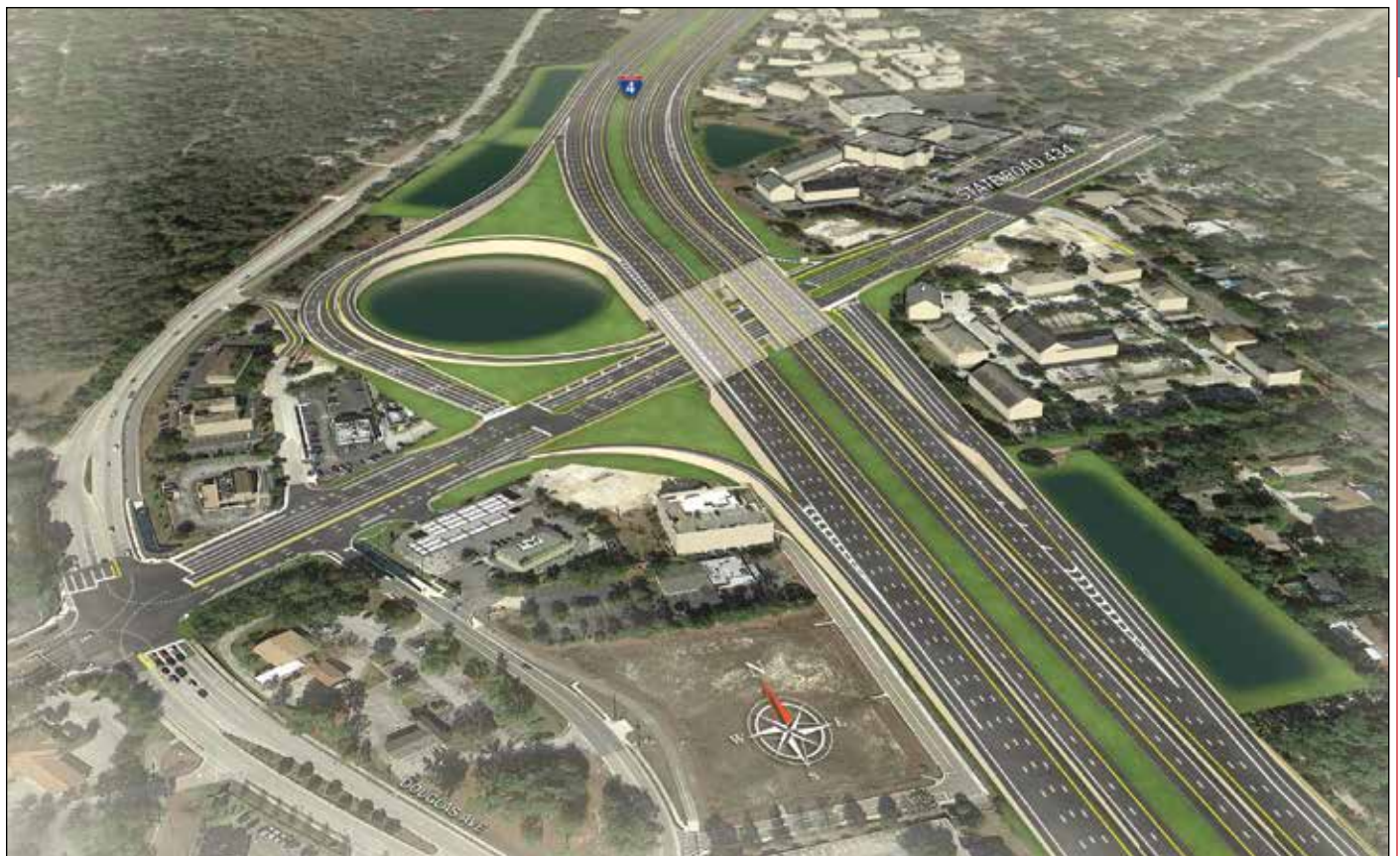
State Road 434 / I-4 Interchange
